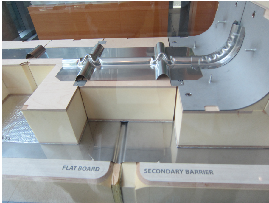
Figure 10: Close-up of insulation in LNG tank
